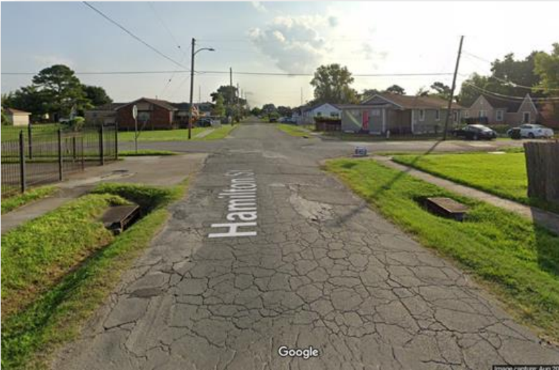
Existing asphalt conditions on the 3000 block of Hamilton Street
