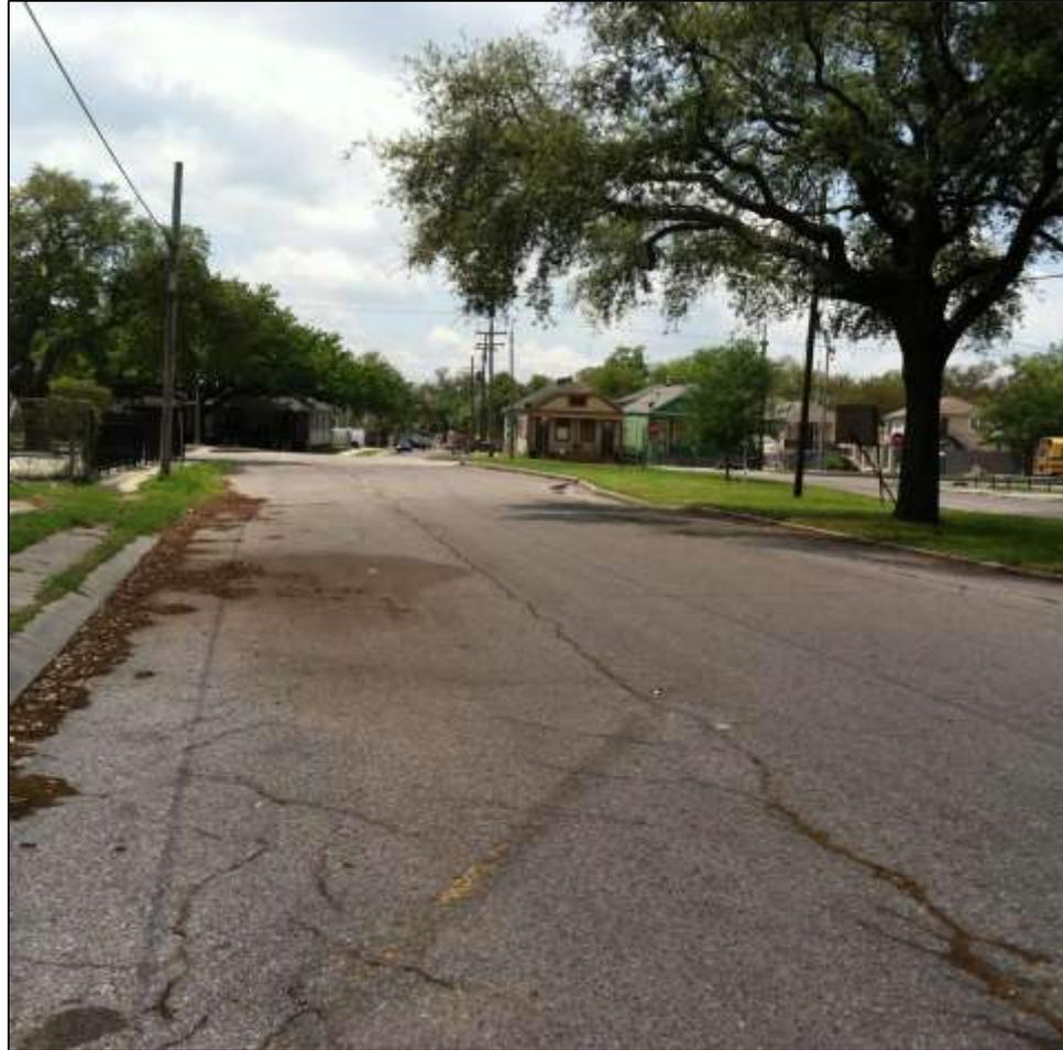
Existing conditions of S. Galvez St. yields a Pavement Condition Index score of Very Poor
