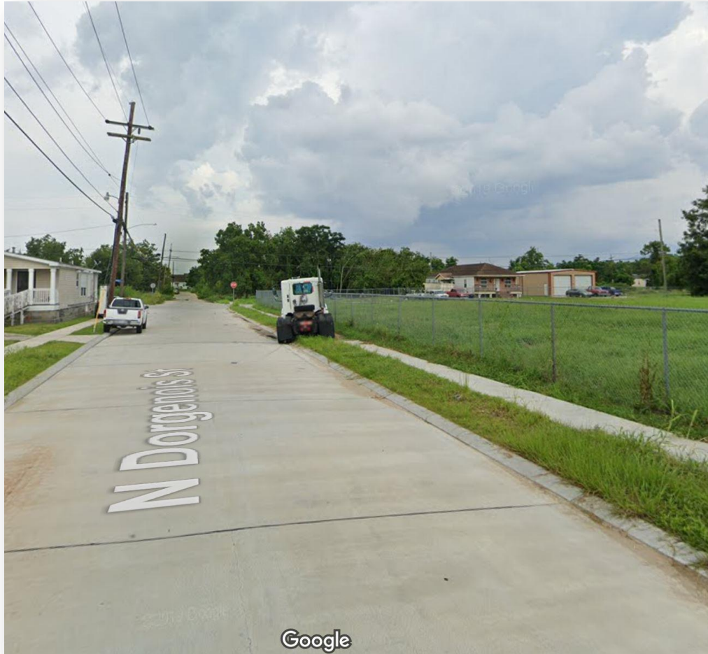
An example of a repaved area of N. Dorgenois St. from the recently completed Lower Ninth Ward Northeast Group A Project.
