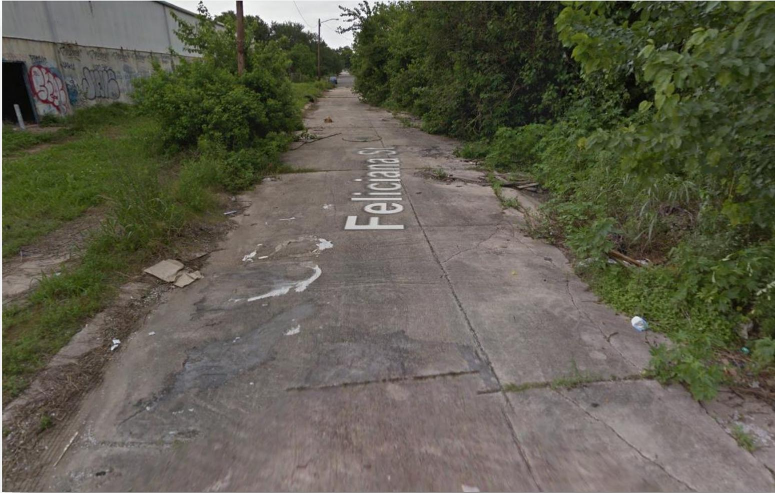
Existing condition 2800 block of Feliciana St. – Pavement Condition Index - Very Poor
